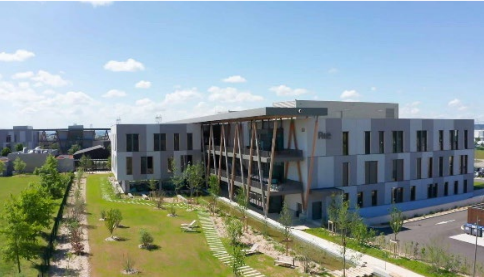
Aerial view of RTE international's laboratory
